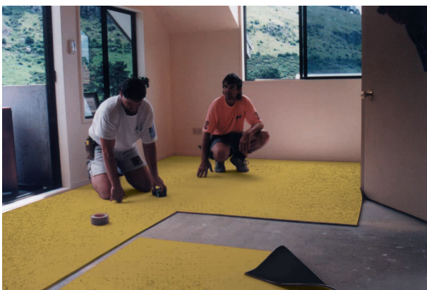
dBX Carpet Underlay, laid using standard installation techniques
